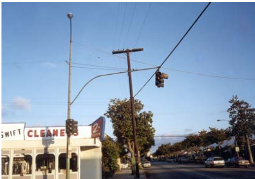
Culver City manually-built mastarm on Washington Boulevard Graphic - 3109
