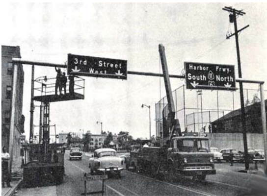
Overhead guide sign on 3 rd Street, circa 1957
