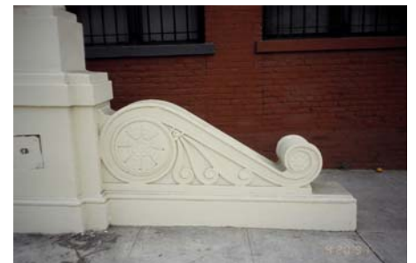
1 st Street bridge over the Los Angeles River
