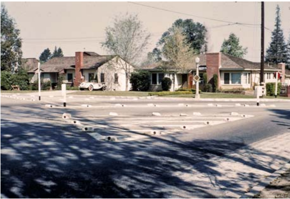
"Metal Mushrooms" used to delineate a flush island
