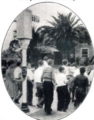
Pedestrians can now act as their own traffic officers with the invention of a new street crossing device by Ralph Dorsey, Los Angeles traffic signal engineer, which is now being tried out. Operated by a push-button, this work-it-yourself signal halts traffic with stop arm and red light for 15 seconds, giving the pedestrians time to cross the street, then it automatically reverts to the "clear" position. Twenty-five seconds must then elapse before another pedestrian can again halt traffic. Photo shows pupils from the Luther Burbank Junior High School in Los Angeles operating the new device.
