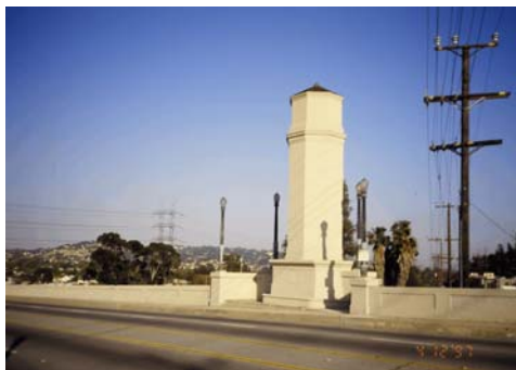
Hyperion Street bridge over the Los Angeles River
