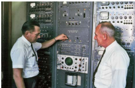
Pro-Rata system in Room 1200A City Hall Graphic - 3010
