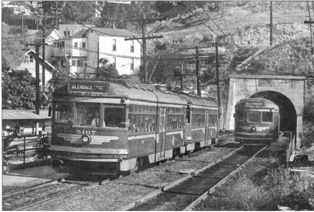
Red Cars and the 1925 tunnel portal southeasterly of the intersection of 2 nd Street and Lucas Avenue
