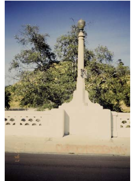
Avenue 60 bridge over the Los Angeles River
