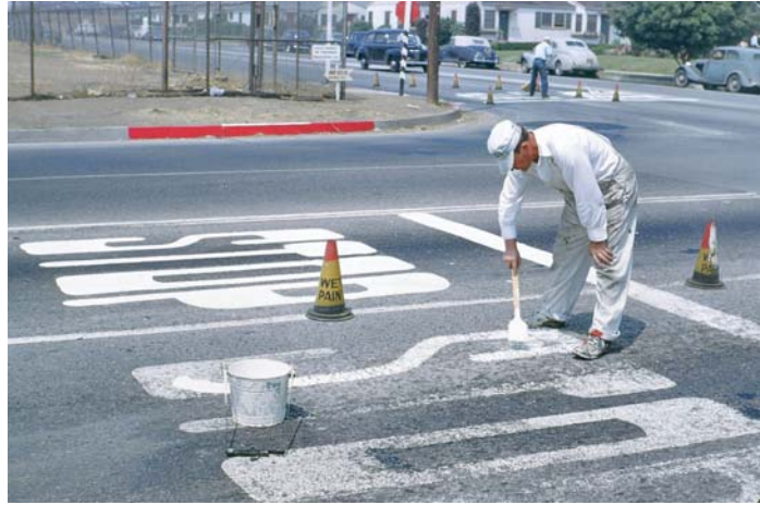
Pavement message maintenance using a brush, circa 1950
