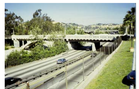
Avenue 26 bridge over the Arroyo Seco
