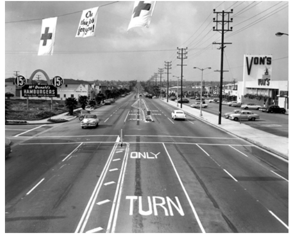
La Tijera Boulevard near Knowlton Street, looking south, March 1956 Graphics - 3058
