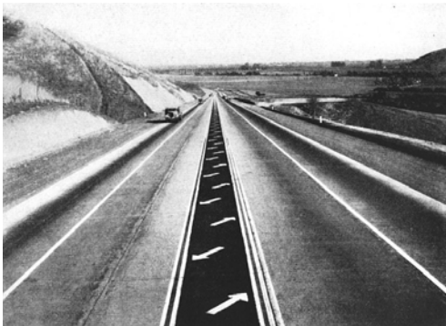
Asphalt-formed diagonal arrows used to separate opposing flows
