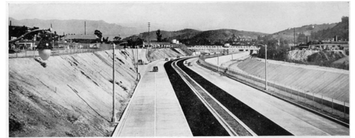
The same spot today looking north from Avenue 26 Bridge.
