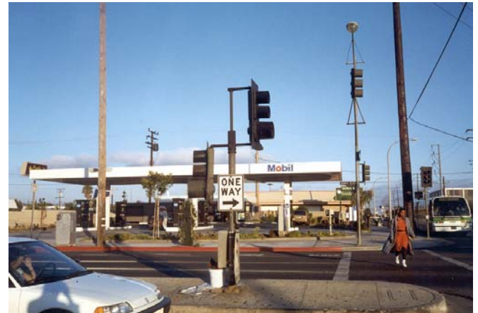
Median-mounted left turn signals before long mastarms became available Graphic - 3112
