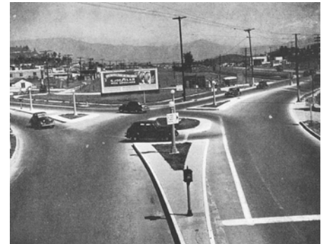
Channelization and markings at the "Y" intersection of Alhambra Avenue and Valley Boulevard
