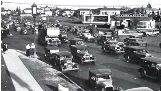
Wilshire Boulevard at Western Avenue, 1929 Graphic - 1023
