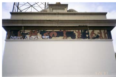
Washington Boulevard bridge over the Los Angeles River
