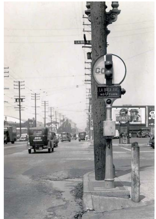
"Waterhouse", the vintage signal of the County of Los Angeles on Santa Monica Boulevard at La Brea Avenue Graphic - 1025
