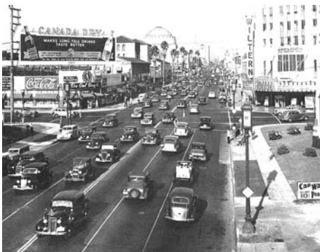
Wilshire Boulevard at Western Avenue, 1937 Graphic—5037
