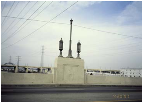
7 th Street bridge over the Los Angeles River
