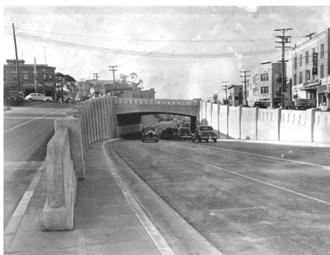
Construction of the Figueroa Street grade separation and diamond interchange at Temple Street.
